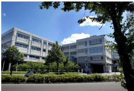
Figure 2 – West facade of Erasmus MC Sophia complex in Rotterdam.
